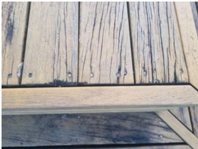
Timber deck to front is showing signs of deterioration
