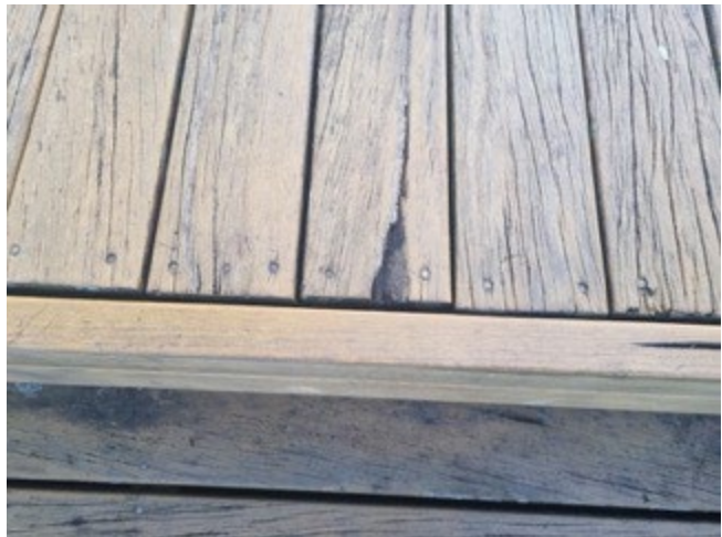
Timber deck to front is showing signs of deterioration
