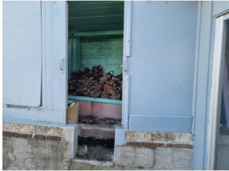
Decorative Plywood enclosure for firewood is rotting in parts
