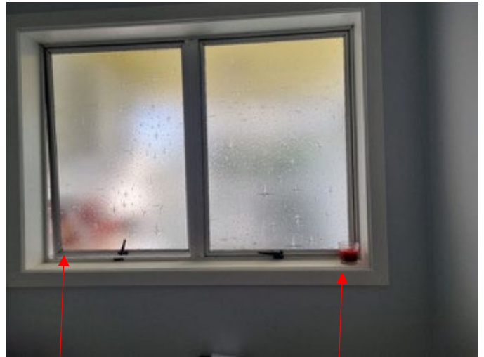
Joinery windows in ensuite & main bathroom are having trouble opening/closing
