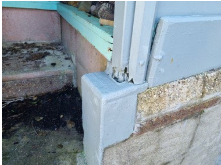
Decorative Plywood enclosure for firewood is rotting in parts
