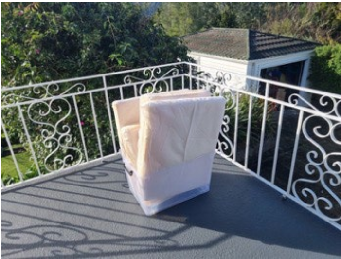
Deck handrail does not comply to today's building standards due to its low height, however it would of complied at the time if consented
