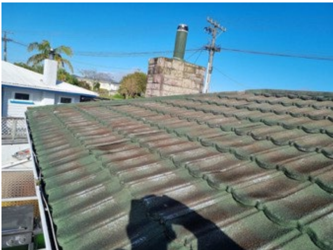
The decramastic roof tiles are due for maintenance (recoating)
