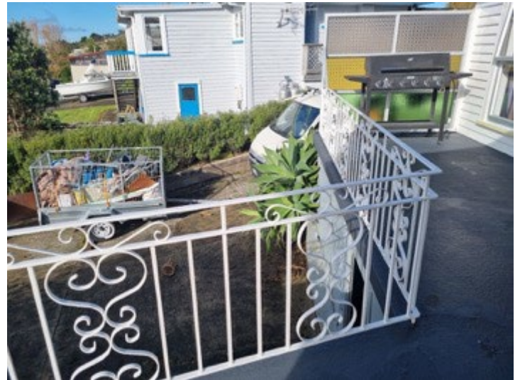
Deck handrail does not comply to today's building standards due to its low height, however it would of complied at the time if consented
