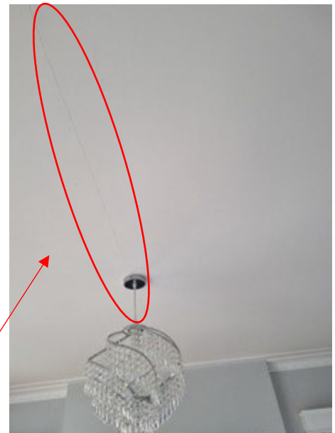
Ceiling has minor cracks in the fibrous plaster throughout due to possible movement over the years
