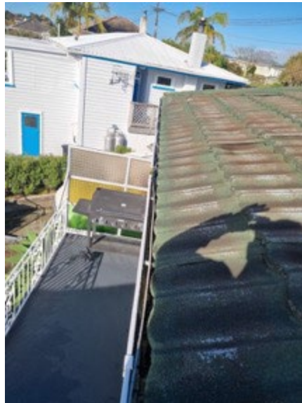
The decramastic roof tiles are due for maintenance (recoating)
