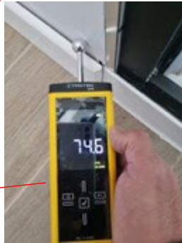
High moisture reading
