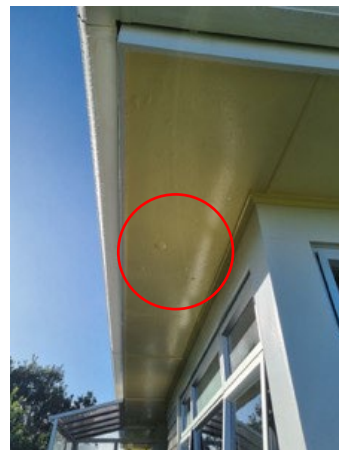
Paint is bubbling in soffit in a couple of areas as per photos
