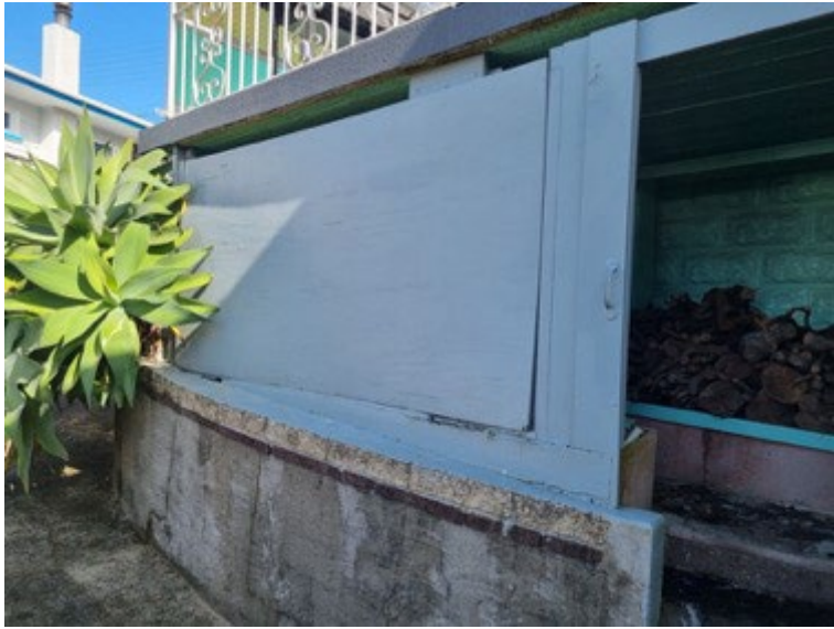
Decorative Plywood enclosure for firewood is rotting in parts
