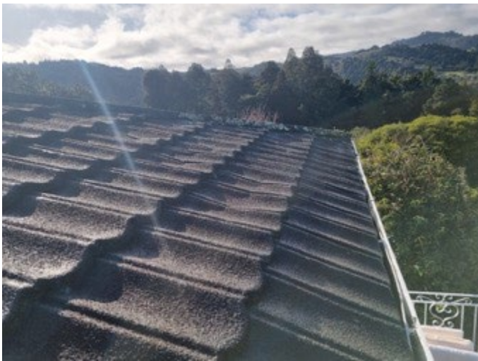
The decramastic roof tiles are due for maintenance (recoating)
