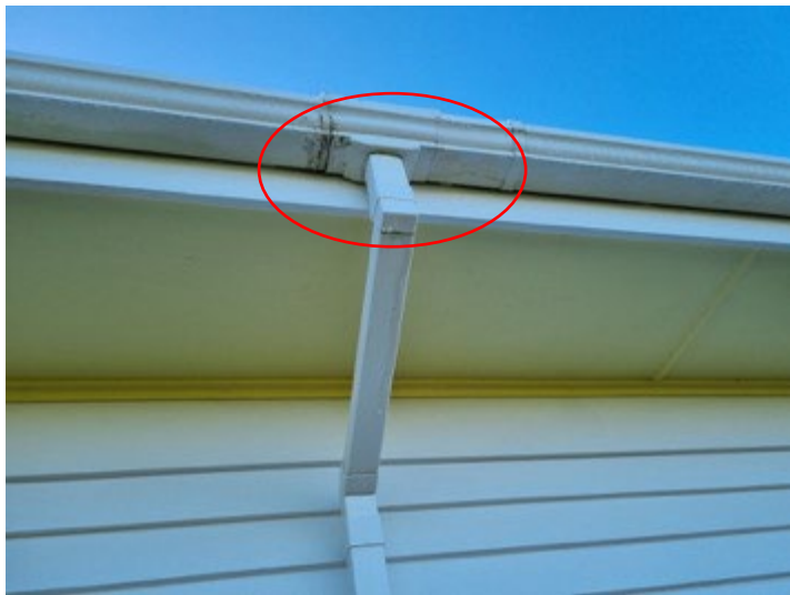
Westside of the house the roof spouting has leaky junction
