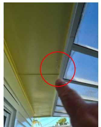
Paint is bubbling in soffit in a couple of areas as per photos
