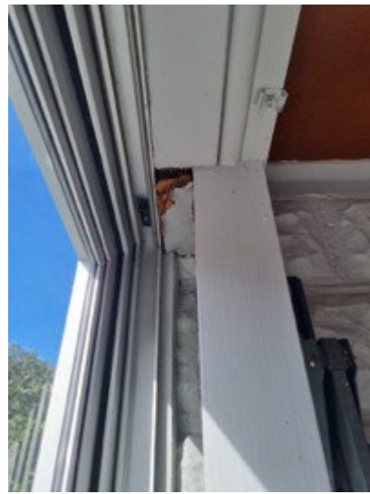
Room off laundry with tiled floor and aluminium joinery, has damaged linings and high moisture meter reading
