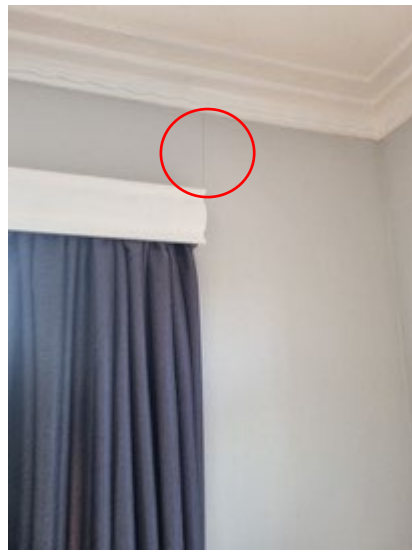
Walls has minor cracks in the gib (or alike) through out
