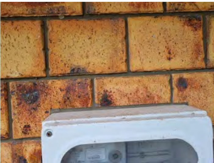
Meter box outside needs sealing and has no head flashing
